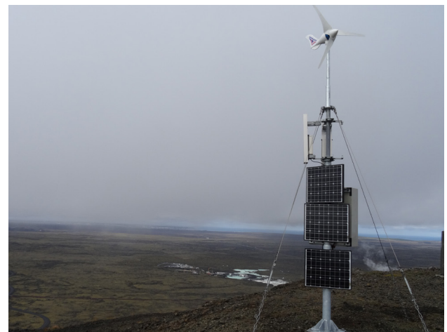
Seismic Monitoring System
