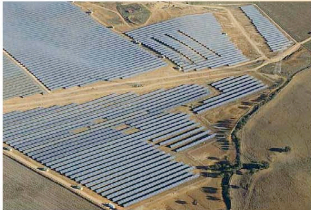
11.48 MW Installation in Valverde de Mérida, Spain
